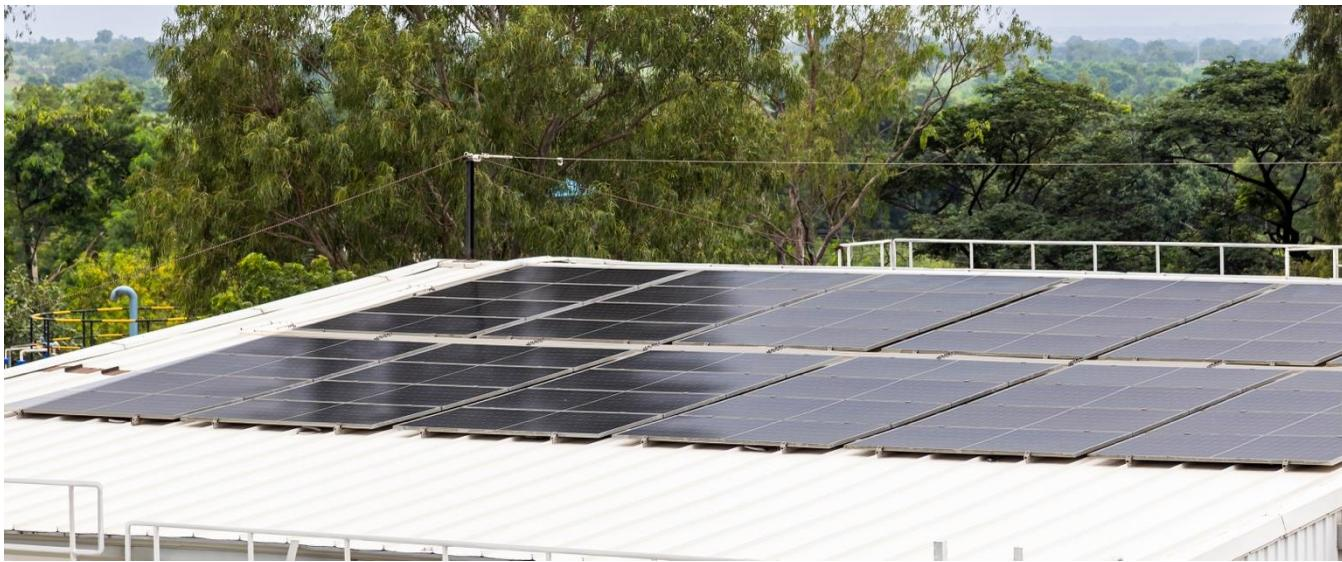
**Digwal (Installation of Rooftop Solar System):** A 240 kWp rooftop solar system was installed in April 2024 to support on-site renewable energy generation. In FY2025, the system generated approximately 607 GJ of renewable power, contributing to a reduction of 123 tCO<sub>2</sub>e emissions. This initiative strengthens our efforts to expand clean energy use within our operations.
